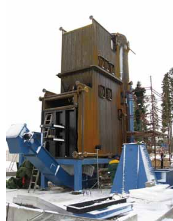
Lapinlahti Ekolämpö 2007, 3,5 MWth waste fired grate boiler
