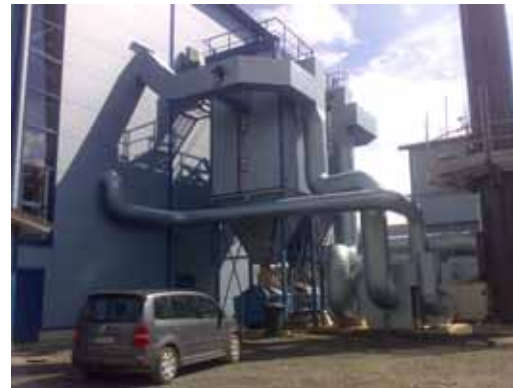
Lapinlahti Ekolämpö 2007, 3,5 MWth waste fired grate boiler
